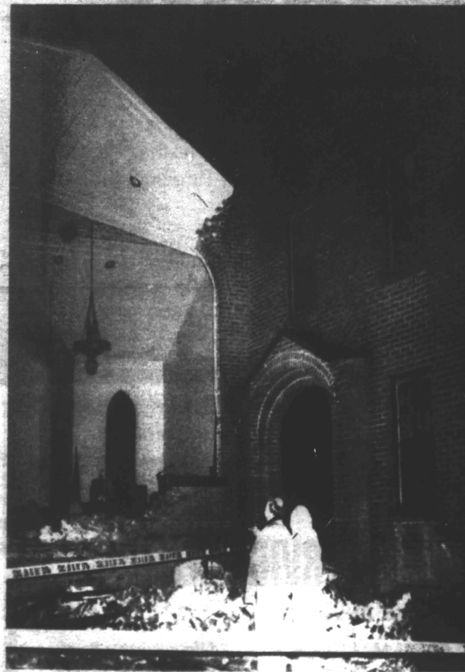
THE REV. RANDY JETTON looked over the heavily damaged First United Methodist Church he has pastored for six years after the storm raged through Halls Sunday. "This open space is where beautiful, majestic stained glass windows adorned the sanctuary," he said.
